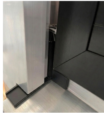
JSCFL-22 - Head and sill cutting before fitting J42/TMT42
