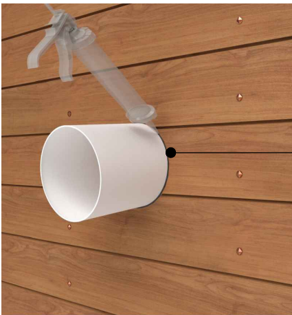
Continuous weather seal around pipe
