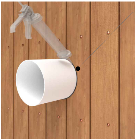
Continuous weather seal around pipe
