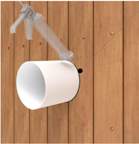
Continuous weather seal around pipe
