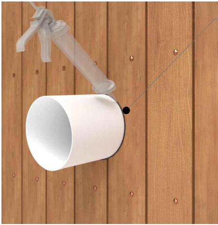
Continuous weather seal around pipe
