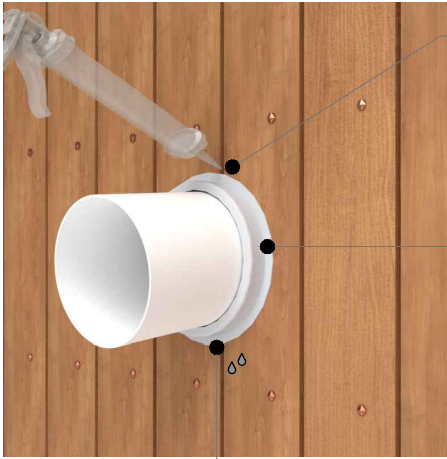
No sealant to drain
