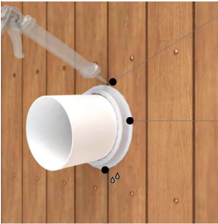
No sealant to drain
